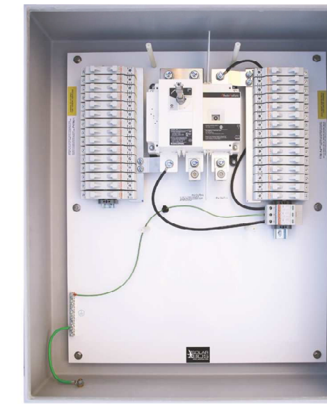
SolarBOS Floating Disconnect Combiner, 1500VDC, 275A disconnect, 15 input circuits, transient surge protection, NEMA-4X fiberglass enclosure
